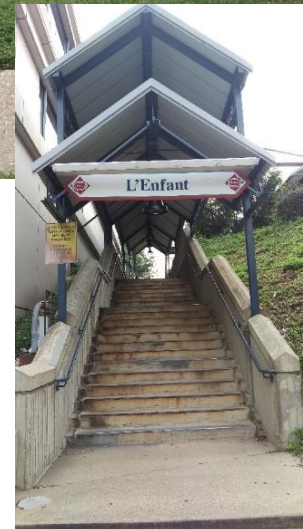
Existing Stairs at 7 th Street SW
